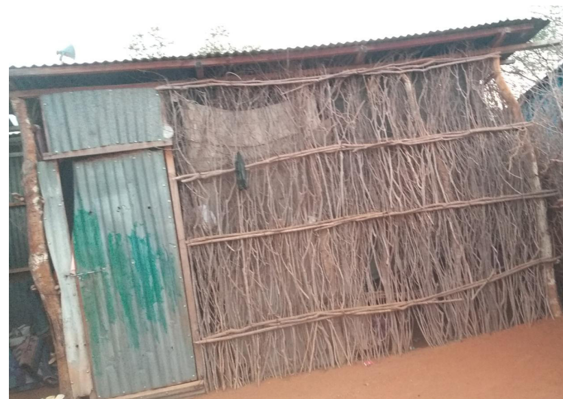
A house made of cordia shrub wall without mud. Photo credit: REACH
